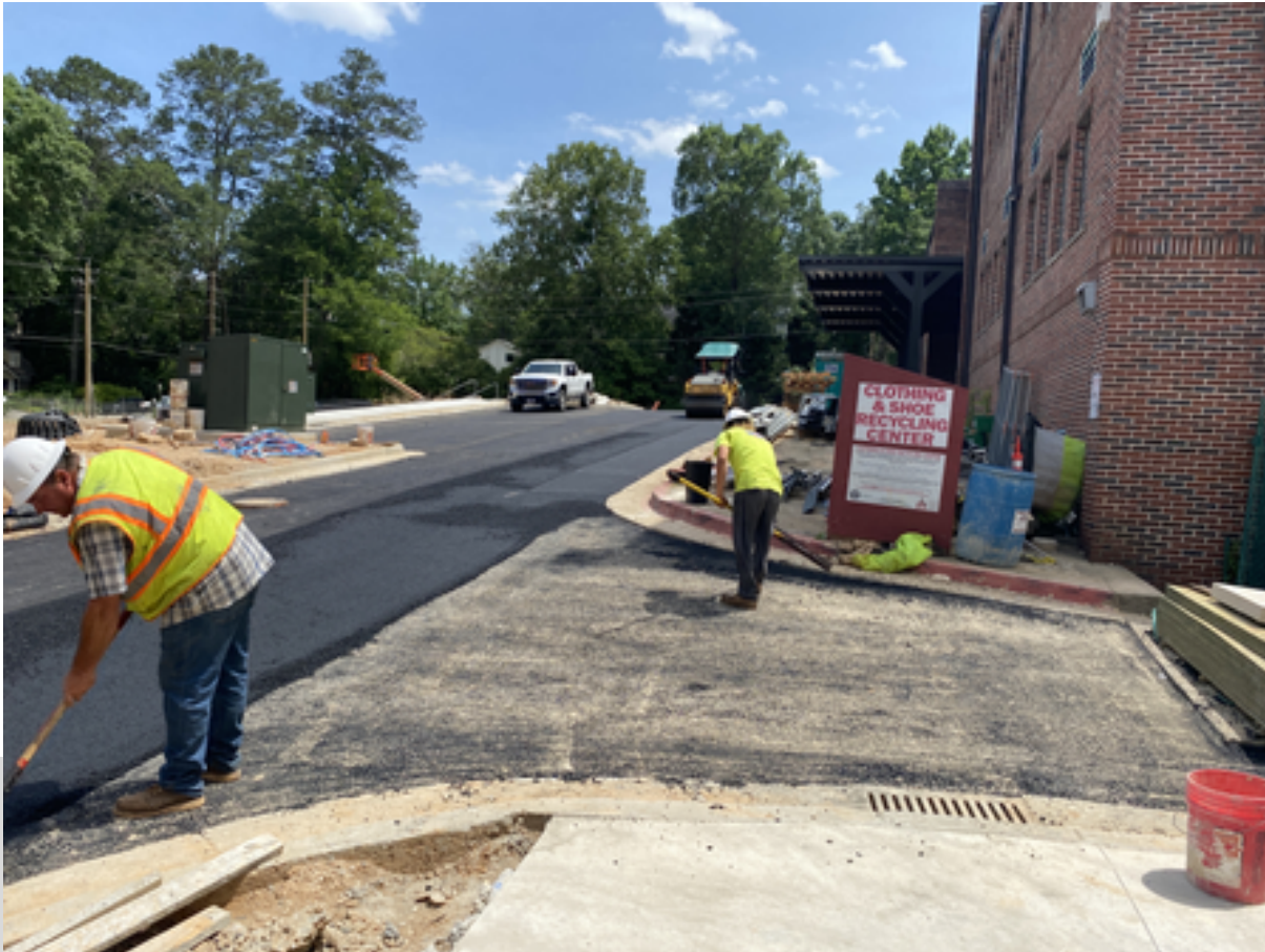
Pavement installation
